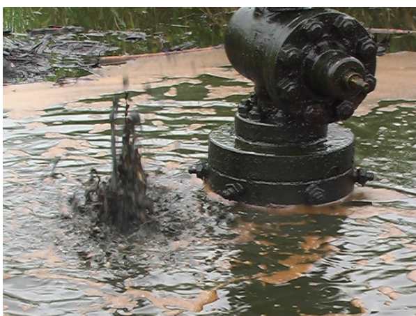
Leaking oil well Photo: Friends of the Earth International
